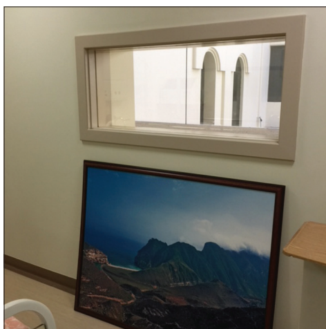
Figure 1: Lead glass window on the concrete wall same size in each of the two rooms
