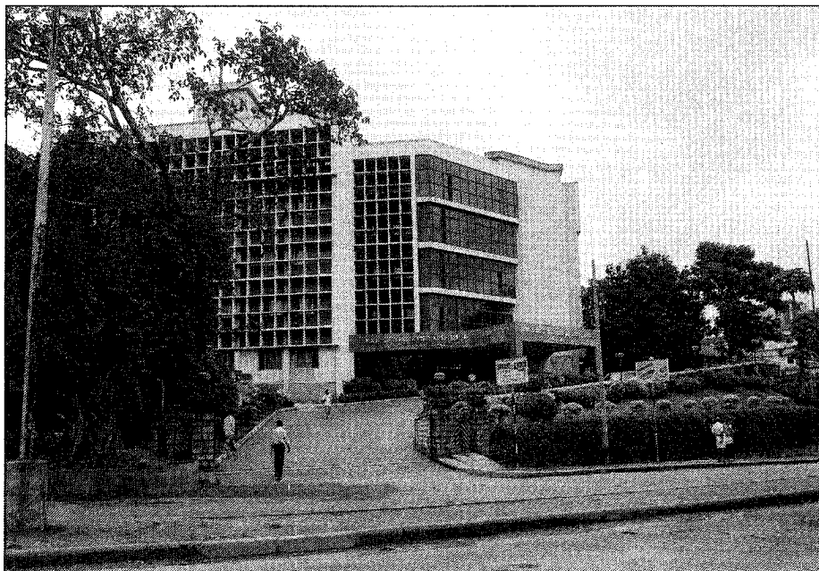
Shirdi Saibaba Cancer Hospital & Research Centre, Manipal
